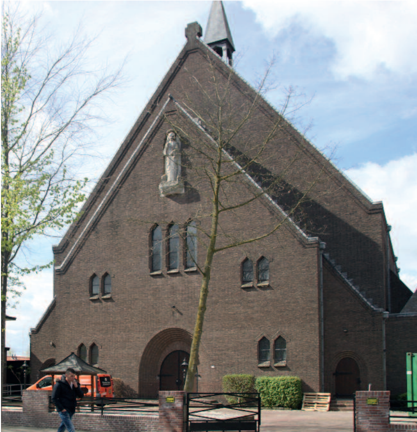
De Vianneykerk, 1929; architect: M. Roebbers
